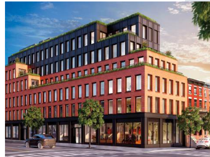
465 Pacific St. | Morris Adjmi Architects
