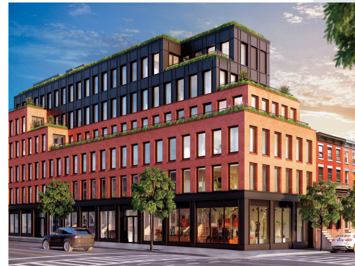
465 Pacific St. | Morris Adjmi Architects
